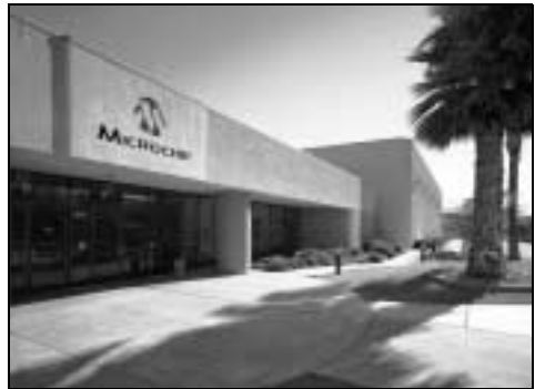
Tempe, Arizona: Microchip's 200,000 square-foot wafer fabrication facility provides increased manufacturing capacity today and for the future.
